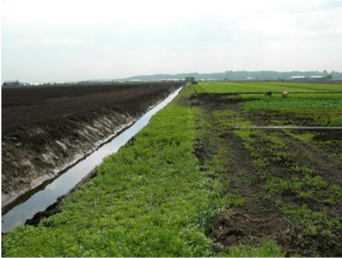
Figure 8: A Typical Dyke and Canal constructed within the Holland Marsh to Control Water Levels
