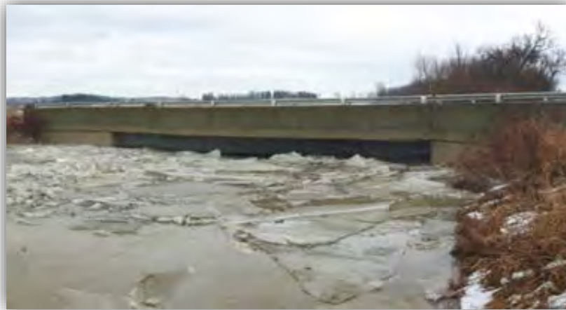
Figure 4-26 Climate change is expected to increase the occurrence of winter flooding.
