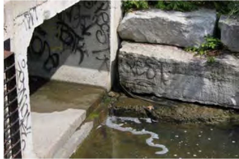
Figure A7.6 : Site 2- Sophia Creek Downstream Side of Culvert
