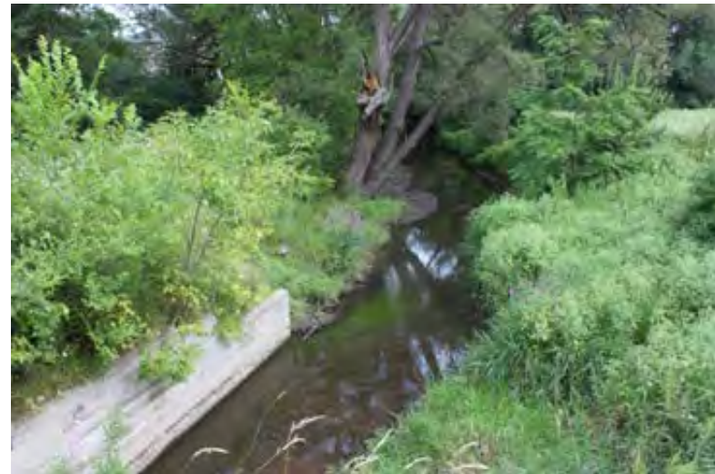
Figure A7. 12: Site 5- Dyments Creek Looking Downstream
