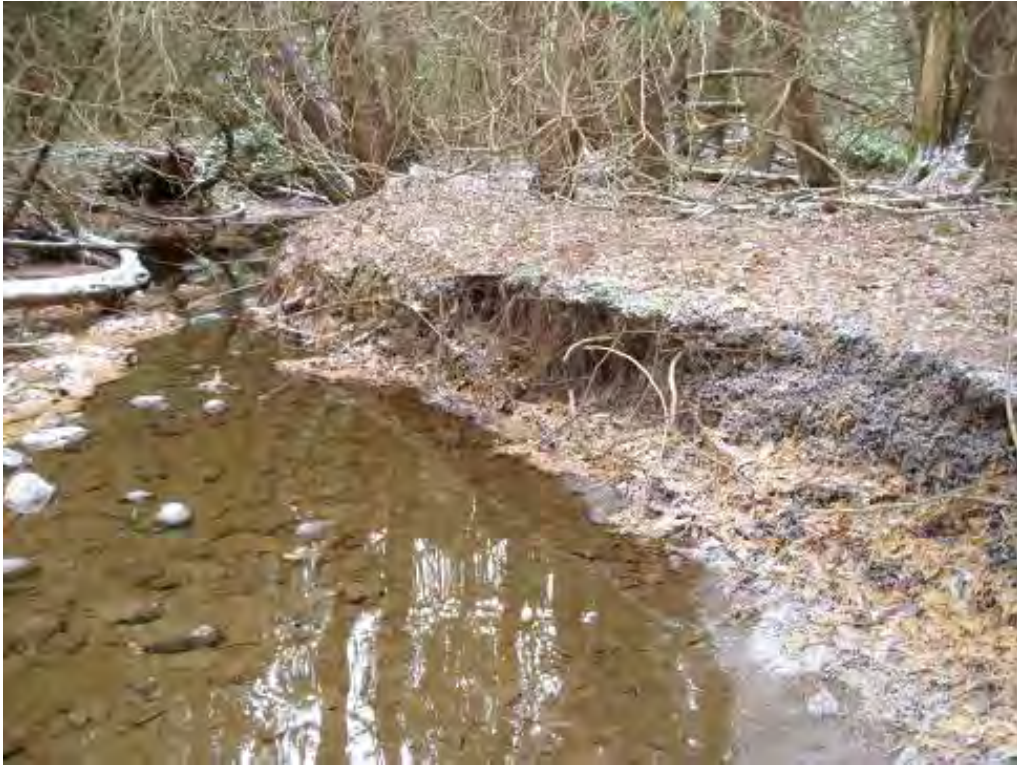
Figure 7-5 Undercutting of the bank (Reach WH 4-8)
