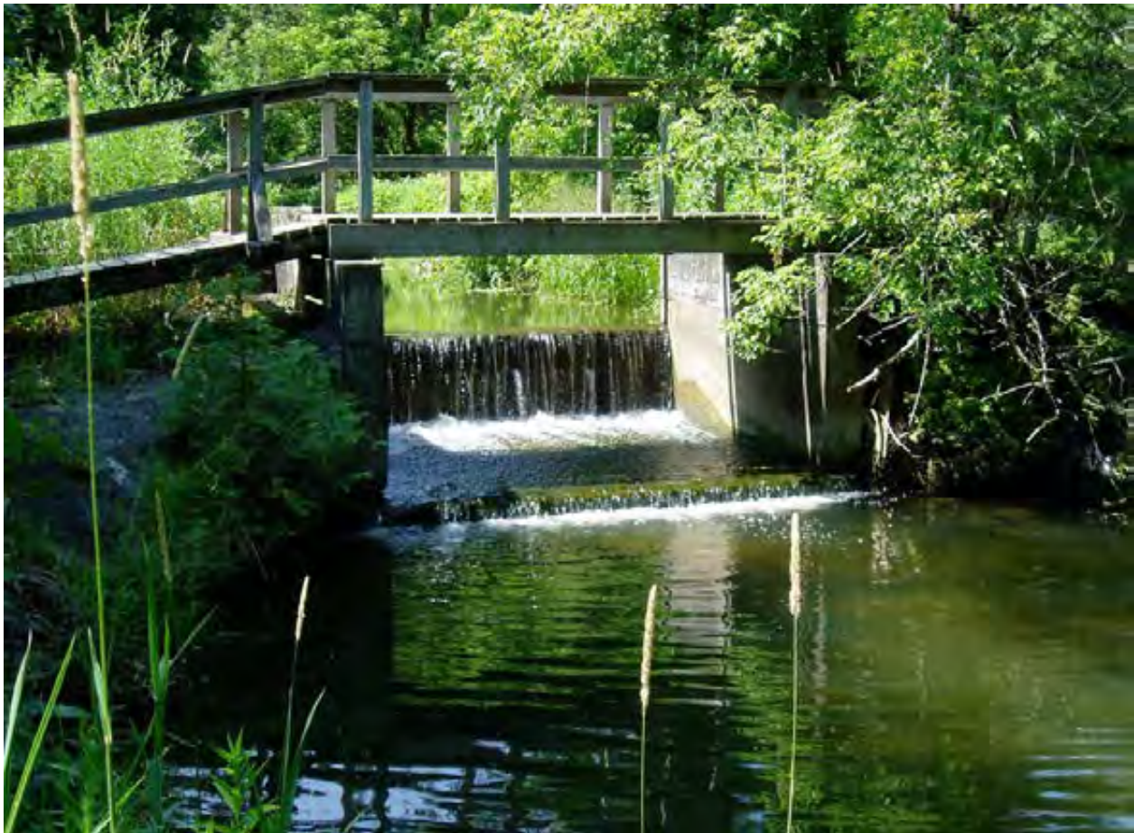
Figure 6-4 The Camp Kettleby Dam – An example of an on-line structure within the West Holland River subwatershed
