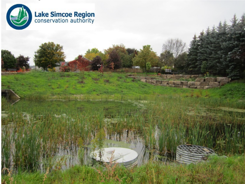
Post Construction of Stormwater Management Pond Retrofit at Colony Trail, East Gwillimbury
