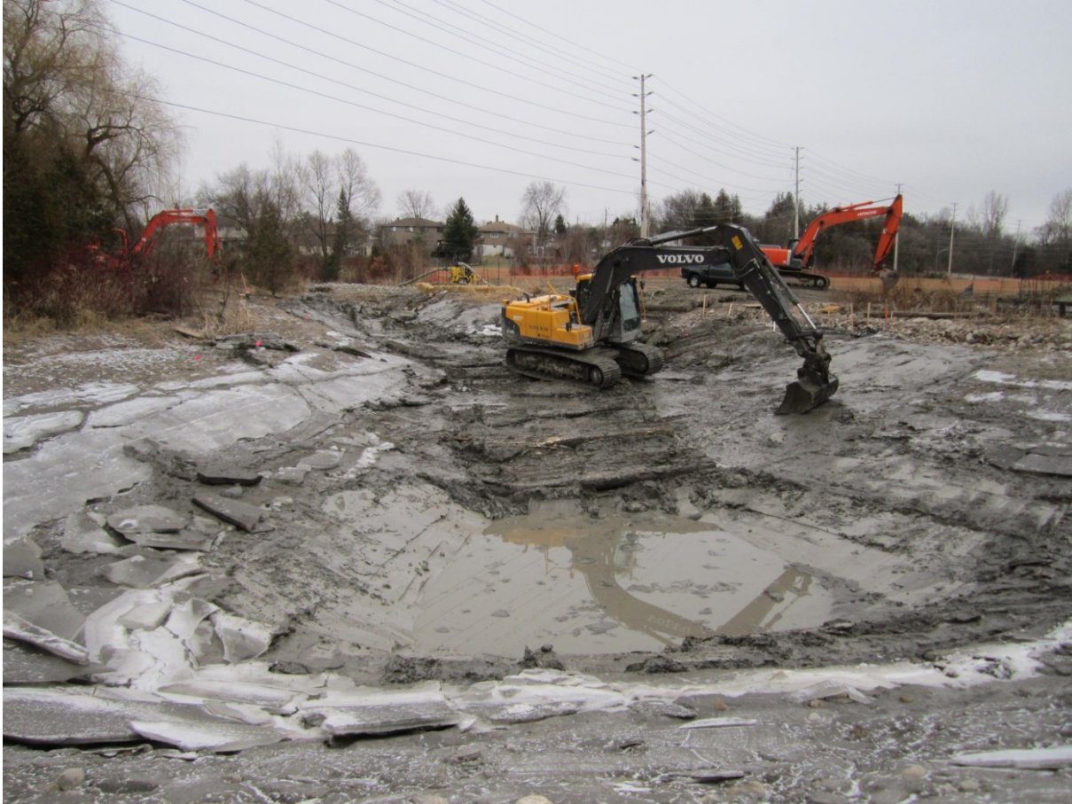
Dewatering and Excavation of Forebay at George Richardson site
