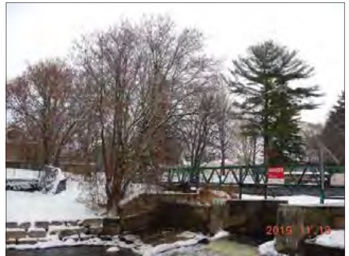
Photo 2702 - Sept 19, 2019 Pefferlaw Dam Large Tree on Right (East) Earth Embankment
