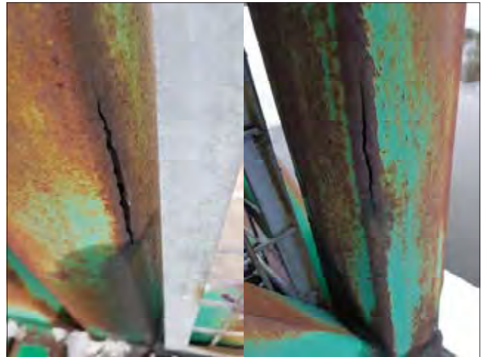
Cracks in Vertical HSS Sections of the Truss Bridge
