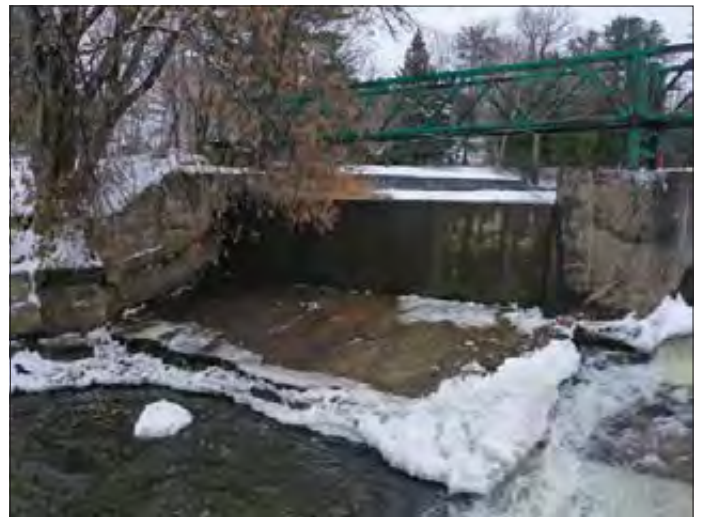
Right (East) Weir, Apron and Dam Abutment
