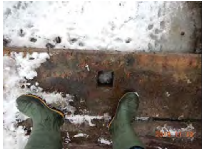
Flashboard Post Hole (Typical)
