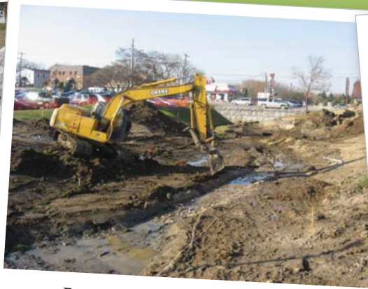
Restoration in process: November 2008
